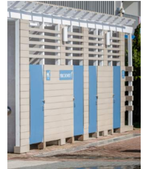
PLASTIC LUMBER ENCLOSURE
